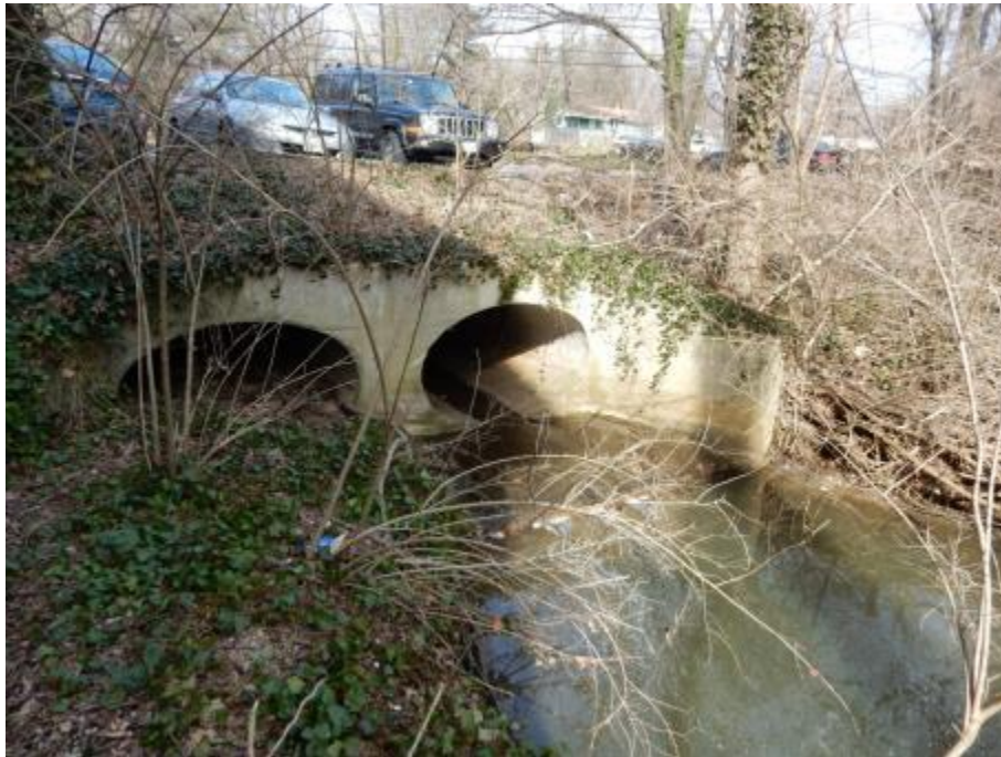
Existing 72-inch RCP Outfalls Crossing Bay Ridge Avenue
